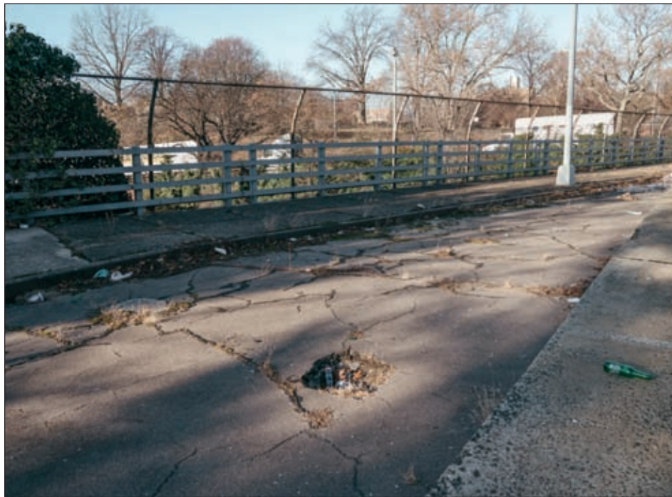
There were visible cracks on the sidewalk on Arthur Avenue overpass along the Cross Bronx Expressway, Dec. 14, 2024.
